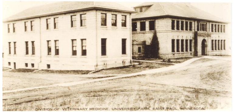
Veterinary Medicine Building (Old Anatomy), right building built in 1901 & left building built in 1915
